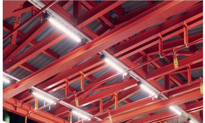
*The luminaires were pre-fitted at the factory with special cables chosen by Borealis.*
